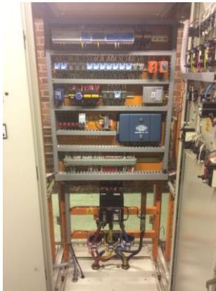
Following the survey it was decided the scope of the works would be to design and manufacture a new “Three” generator synchronising control system.
